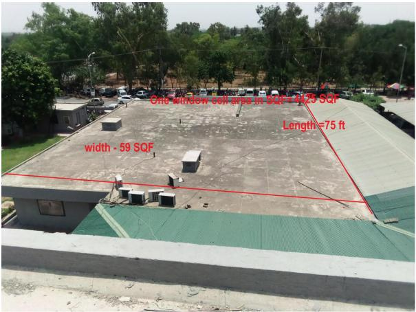
Sanction load of FBISE is 403 KW and one main Transformer of 630 KVA is energizing the whole FBISE Building through a common LV Panel which is 30ft away from Roof areas. During load shedding Diesel Gen-Set is available which will be synchronized with PV System. Please provide complete PV Diesel Synchronization system enabling automatic start of Gen-Set and synchronized operation of PV system with Gen-Set supplying energy to load in safe manner. ATS is already available.
