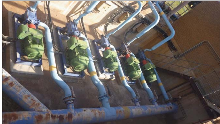
Figure 7-7: Photograph of the Irrigation Pond Pump Station
