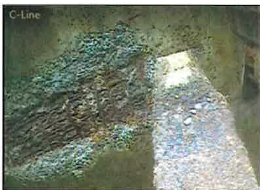
C - Line slab and pile delamination. Group 23
