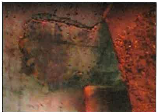
Delamination/Honeycombing B3 - B1
