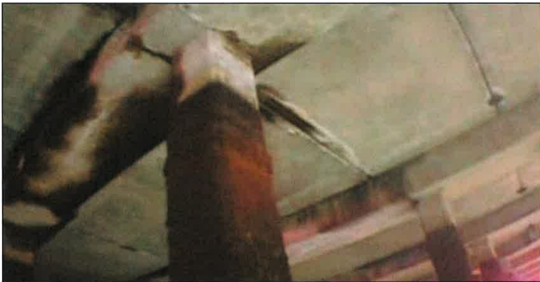
Figure 27: Typical precast deck supported by primary 1000x500 insitu downstand beams
