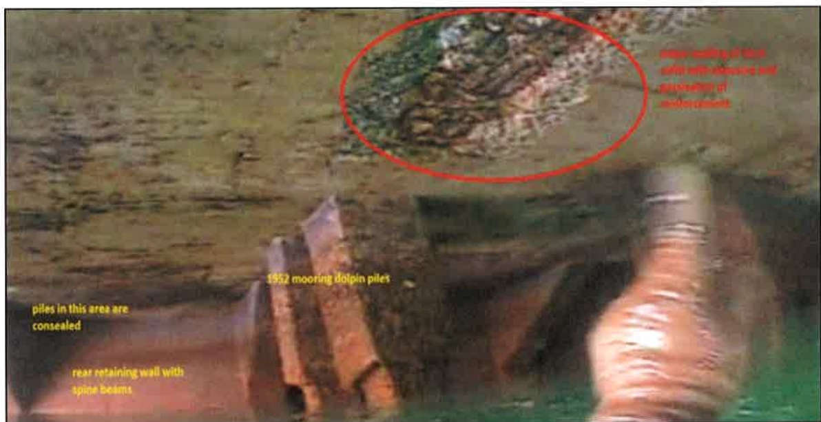
Figure 26: Typical spalling below soffit of old section (1952). Major spalling of concrete and depassivation of reinforcement
