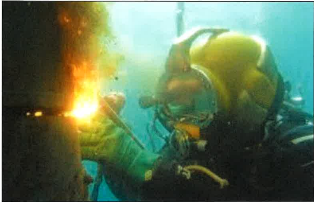
Figure 41: Underwater cutting of corroded rebar
