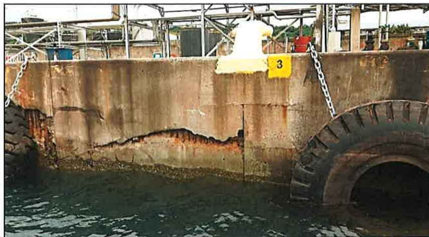
Figure 1: Spalling of concrete on quay wall
