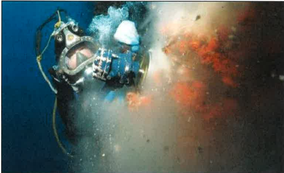
Figure 39: Preparation of underwater concrete structure
