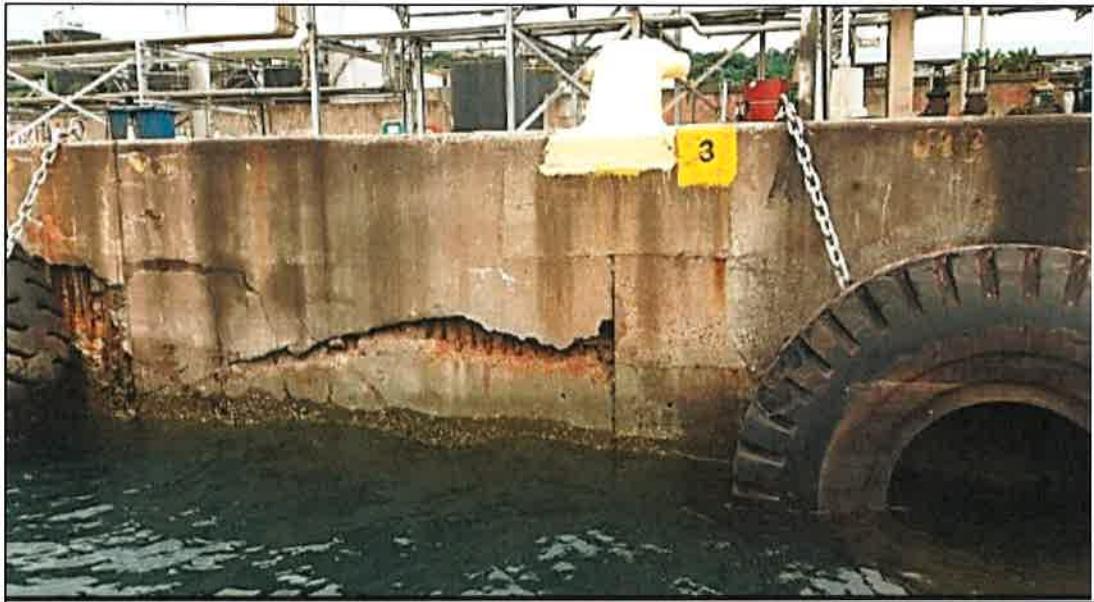
Figure 28: Impact damage on Quay Wall
