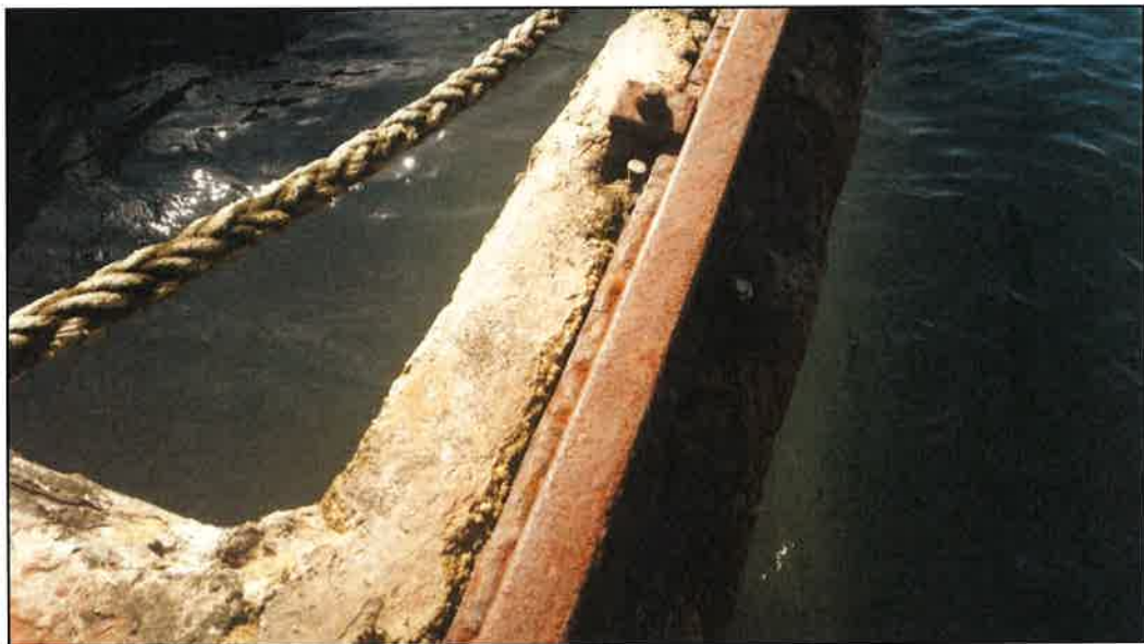
Figure 7: Abrasive damage to concrete structure by wave actions
