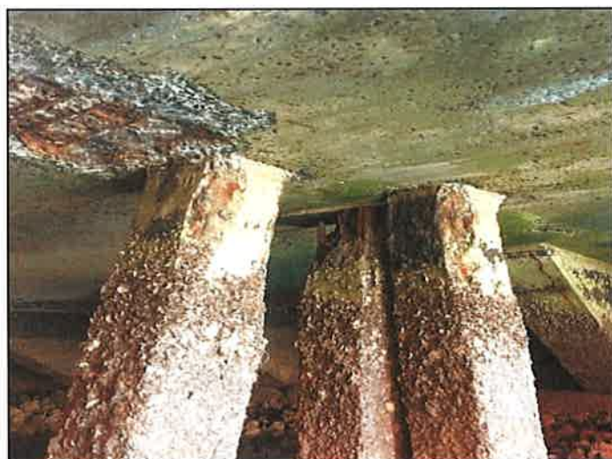
Figure 2: Underdeck concrete spalling
