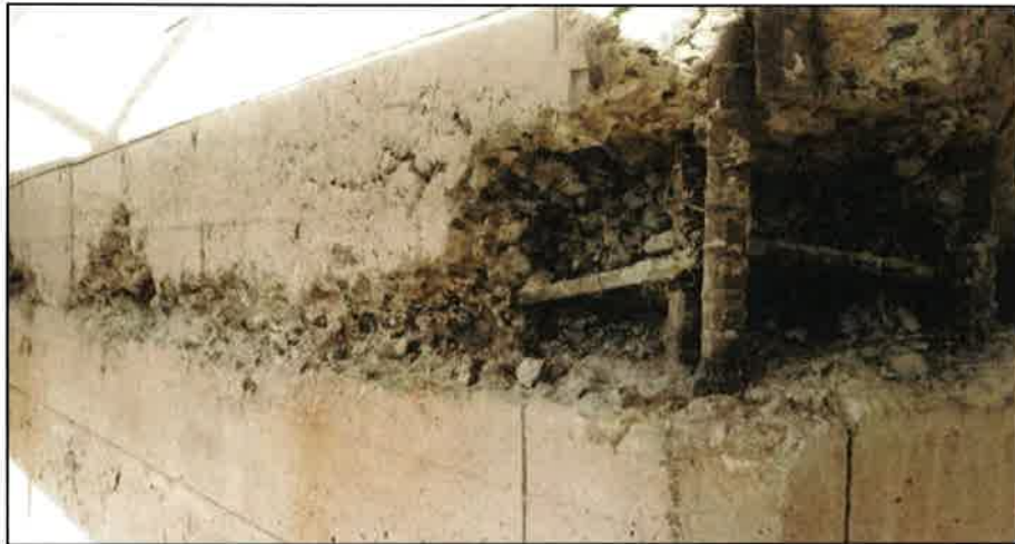
Figure 6: Example of a spalled concrete structure
